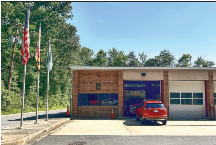
Greenbelt Volunteer Fire Department on Crescent Road
