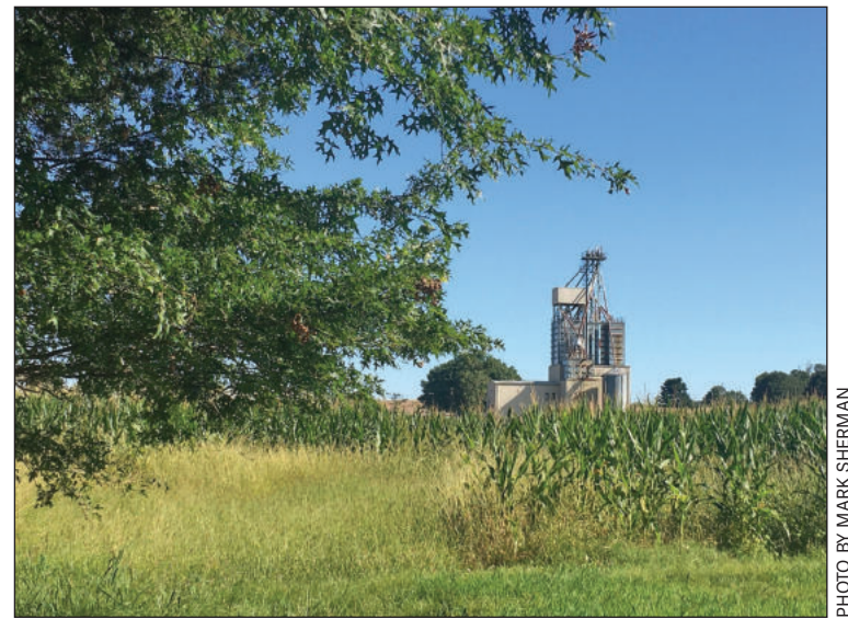
View of BARC on August 30, 2025
