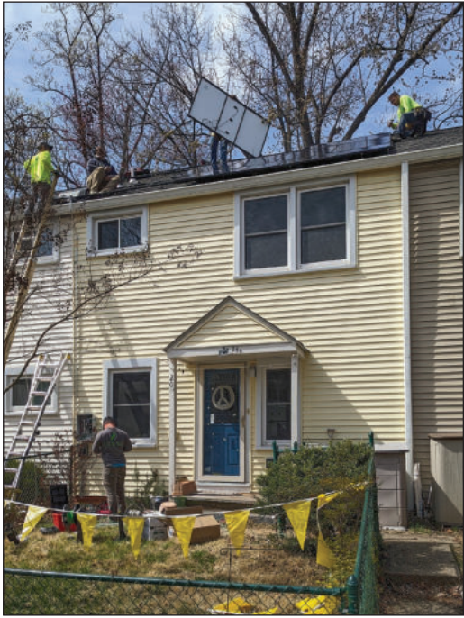
Solar panels are installed on a GHI frame house roof.
