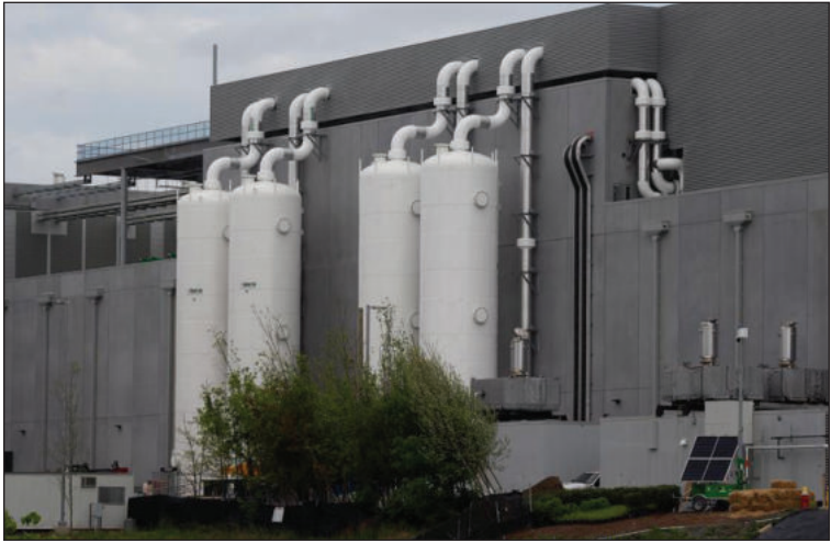
Chilled-water storage tanks are seen on the side of a data center in Loudoun County, Va. Such systems are for backup cooling, according to the company's website.
