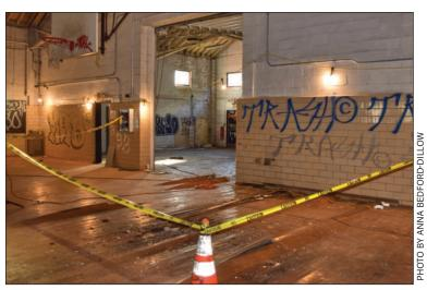
A damaged roof has led to water damage that impacts the ceilings and floors of the Armory.
