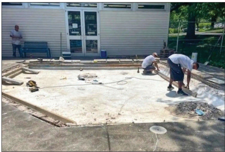
As part of the indoor pool renovations (see story on page 1), the outdoor wading pool is being repaired to fix a leak.
