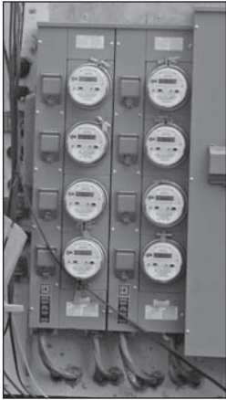
Multiple Smart Meters are located on end units of frame GHI homes.
