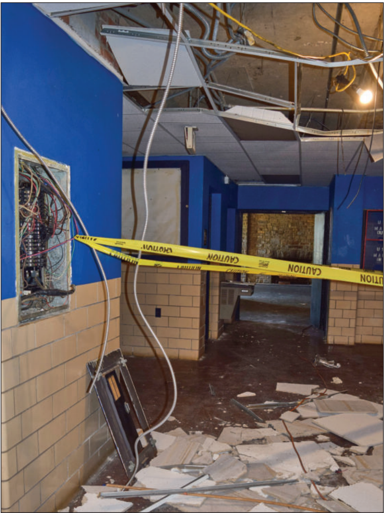
When council toured the Armory building in October, following its acquisition, they found that copper wires had been stripped from electrical boxes, the ceiling was bowed and rubble had filled the corridor.
