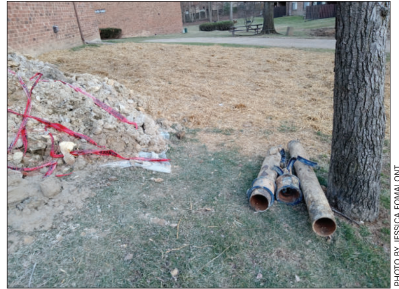
The broken pipes and excavated area are shown after the pipe repair near building 8459 in Chelsea Wood.
