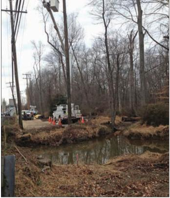
Utility crews relocate overhead wiring along Sunnyside in preparation for a new bridge, bike lanes and more.
