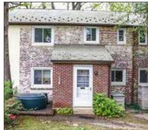
Left: Adding a 9x7 ft. addition to a two bedroom brick home created a powder room, extra storage and a pantry closet. Using the original service side door and matching the brick structure makes this addition blend well with the outside of the unit.
