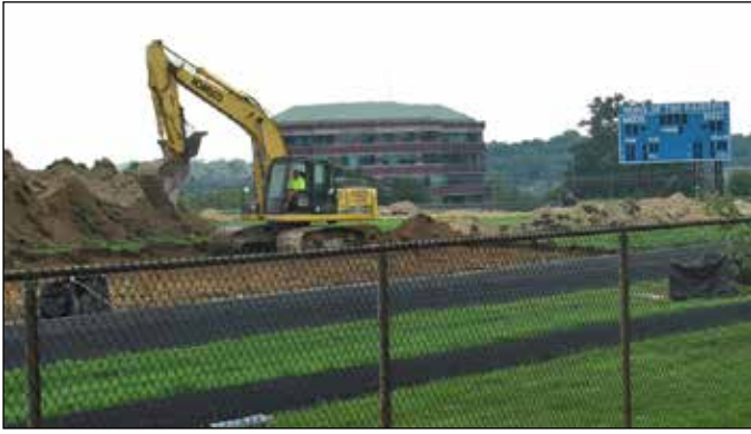
Workers start pulling up Eleanor Roosevelt High School's track on August 2.
