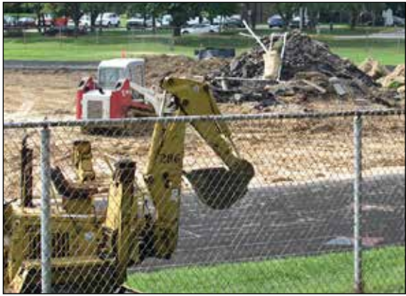
Construction is underway on the ERHS track.
