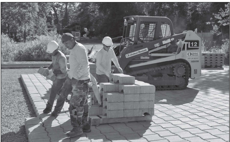
Pervious pavers were installed over a gravel base which allows runoff to filter through.
