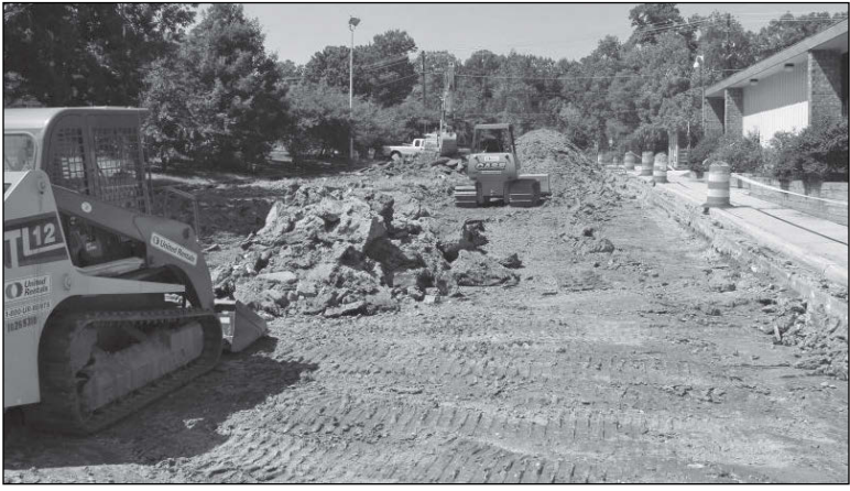
The old asphalt parking lot was completely removed.
