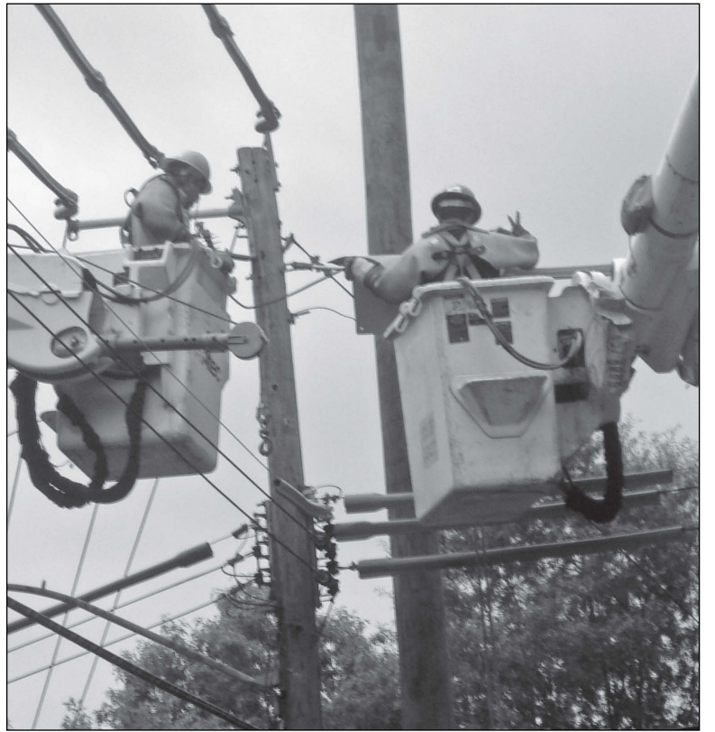
Eddie Rivera (left) and Brian Parks wrap rubber sleeves around the existing primary wire as a safety measure in preparation for "pulling." Existing three-phase wires on existing pole are already wrapped in sleeves. New pole, right, is about 10 feet higher than existing pole.
