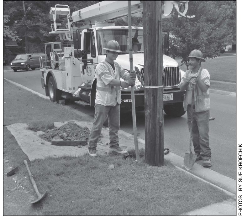
Lucas Preiser (left) hand-digs the hole for a new pole while John Hare waits to remove loosened dirt. The hole needs to be seven feet deep to hold the 45 foot new pole.
