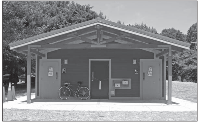
Greenbelt Public Works Department has constructed a new restroom facility at Buddy Attick Park. - photo by Joel Mason-Gaines
