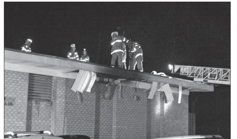
Firefighters found fire showing from the roof of a heating plant.
