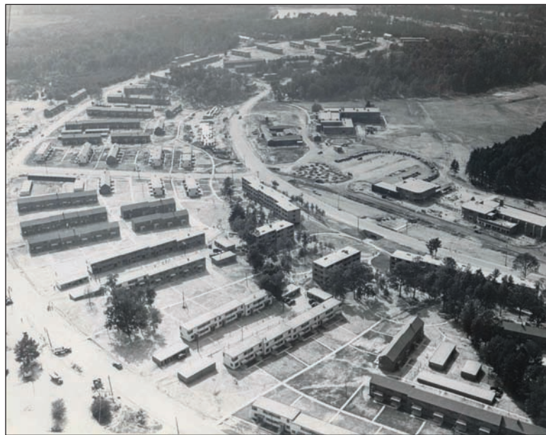
Aerial view of Greenbelt under construction.
