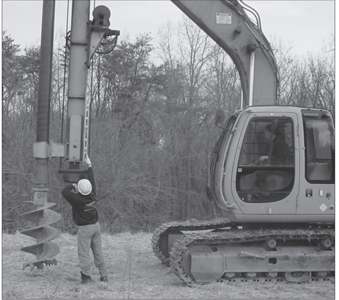
Above, the drill is leveled before every bite.
