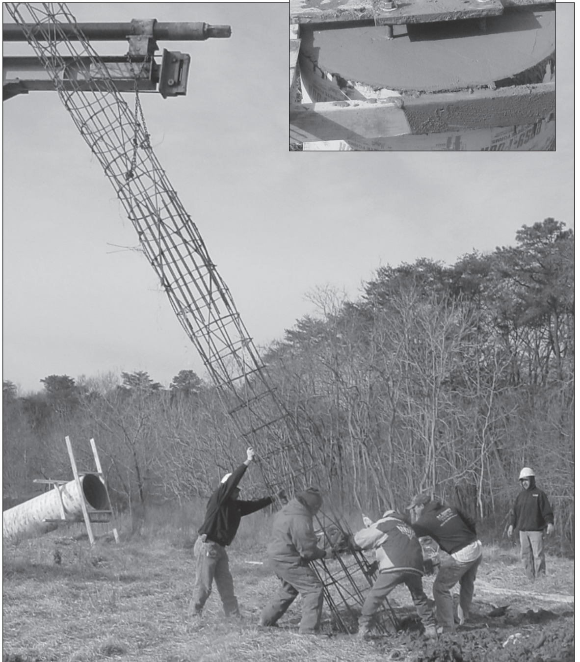
At left, Netsum holds Herman's feet as he unbolts the shovel from the caisson.
