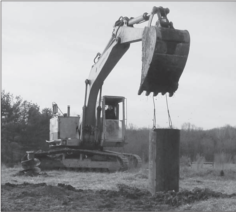
On February 12, a warmly dressed Geo Tech crew set out to install an astronomical pier at the Northway Fields. City inspectors also examined each phase. The pier will support the 13" telescope in the Northway Fields Observatory.
