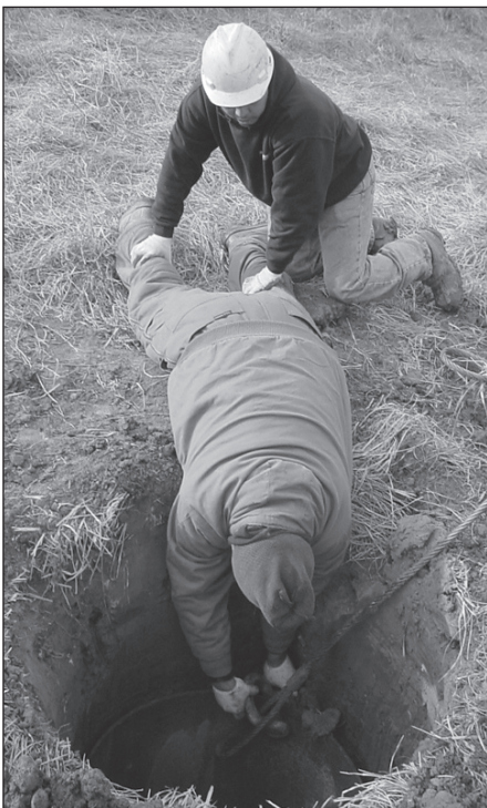
At left, Netsum holds Herman's feet as he unbolts the shovel from the caisson.
