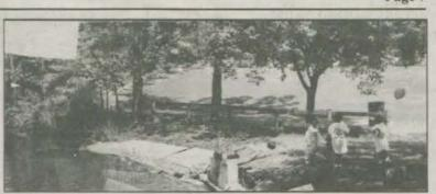
The Greenbelt Lake Shore Restoration Project was a featured part of Greenbelt's Earth Day. The old retaining wall at the bay end of the lake has been removed and the shoreline regraded.
