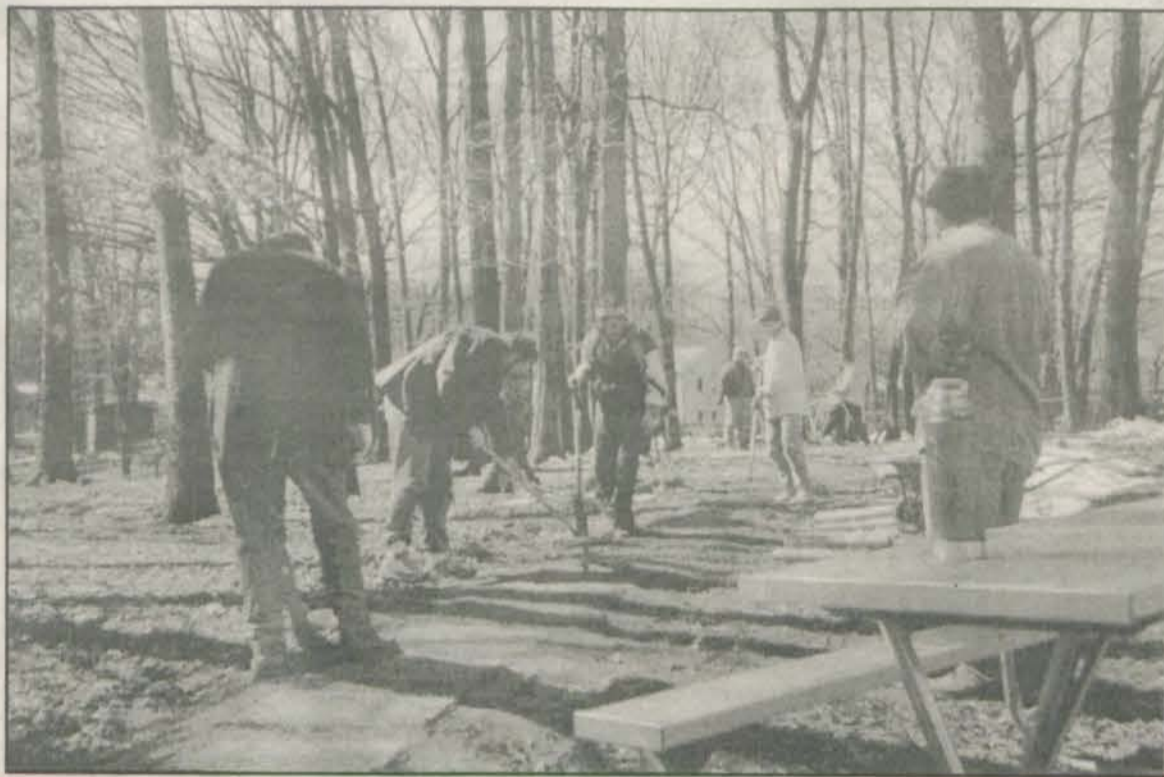
Volunteers lay new flagstone path behind 53 Court Ridge.
