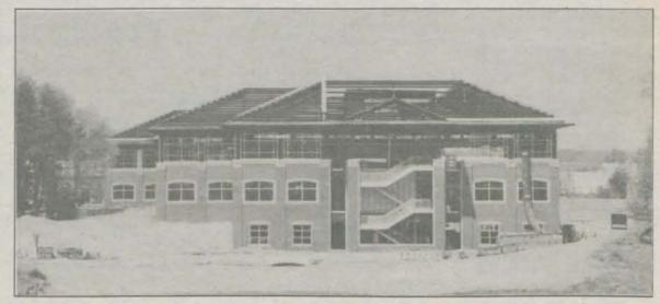
East Wings of Dept. of Agriculture bldg. with brickwork going up as seen from Beltway.
