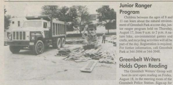
The parking areas around the community center are being reconstructed in preparation for the fall opening of the city facility. Earth moving equipment is being used to remove bad pavement and concrete. A pile of forms for pouring new concrete is in the foreground.
