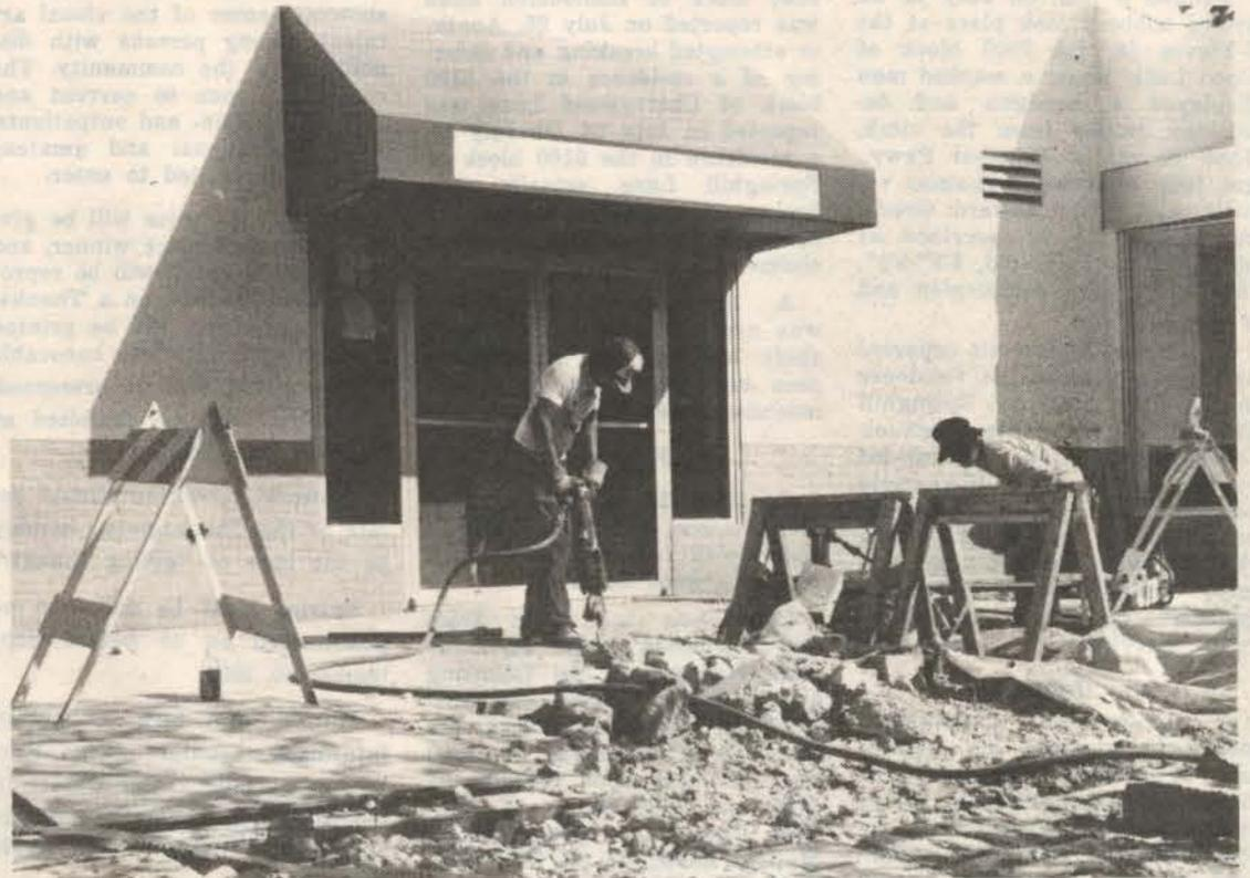
Digging up the sidewalk is one step in installing the ceiling sprinkler system
