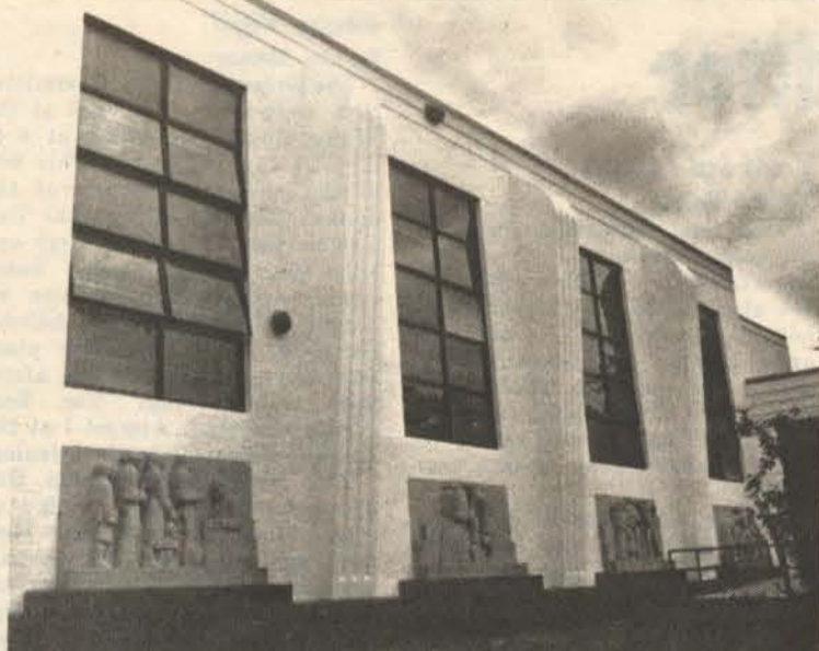
The curved aerodynamic struts contrast with the rectangular windows and structure of Center School. The friezes echo this contrast.
