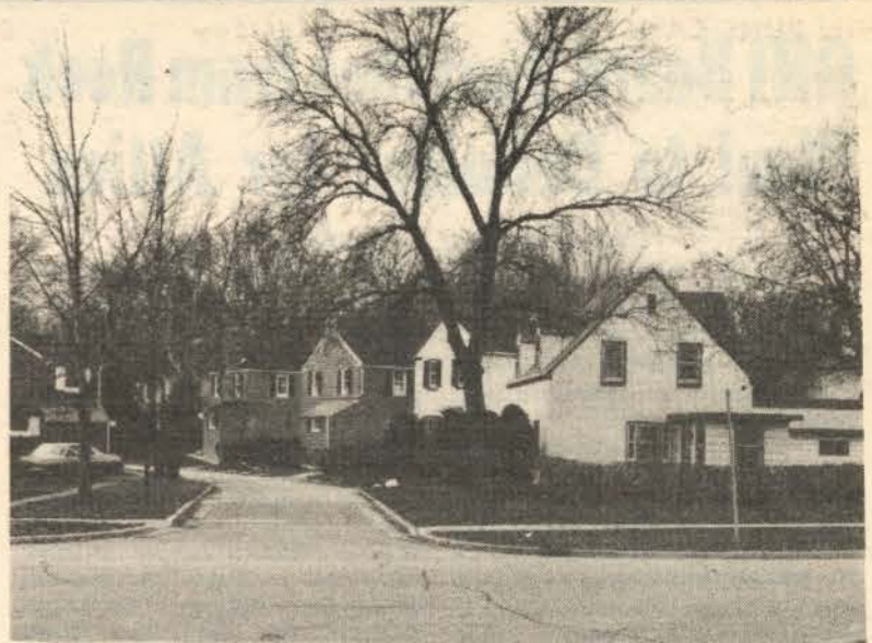
Original free standing houses line a narrow curved street in Greenbelt's sister city, Greendale, Wisconsin. This 1980 photo shows some of the variety present today as owners have added rooms, new siding and shutters or changed the original white color. Houses that come on the market are snapped up quickly. They sell for $50,000 and more.
