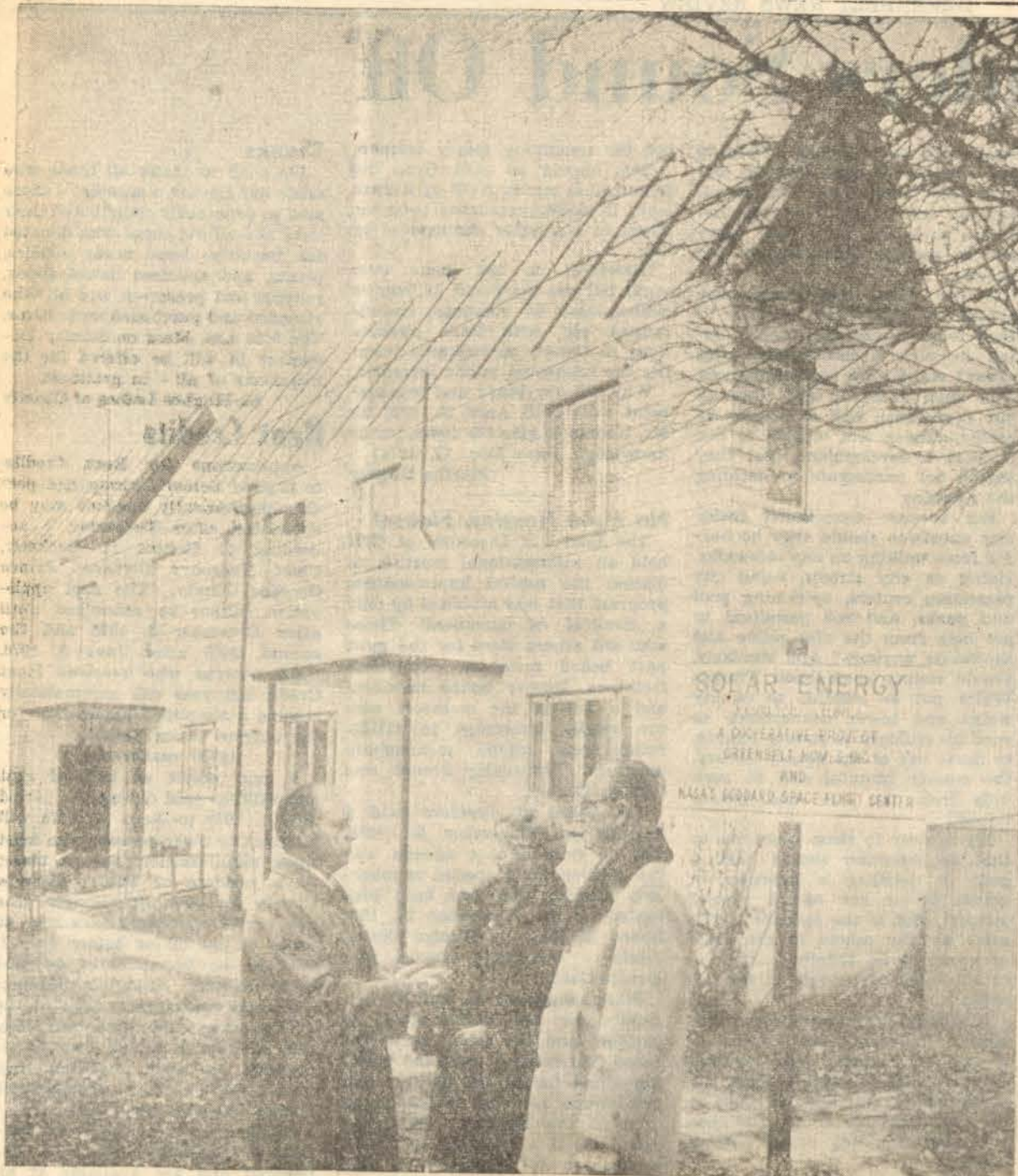
Mr. and Mrs. Joseph J. Karitas of 2-D Southway discuss with Greenbelt Homes, Inc. Director of Maintenance George Craft the adaptation of the solar energy system to their normally flat-roofed home for evaluation during the upcoming winter. The glass-covered solar energy collectors, which are mounted at pitched angles on the roof of house; network of small water pipes affixed to a metal heat absorber.
