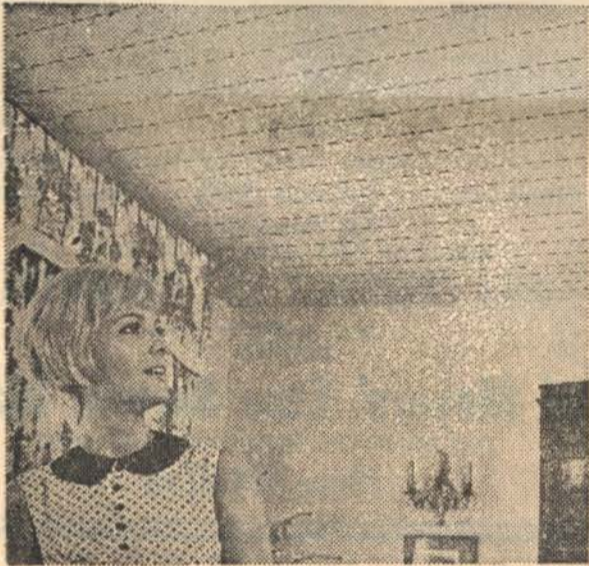
Electric ceiling cable
