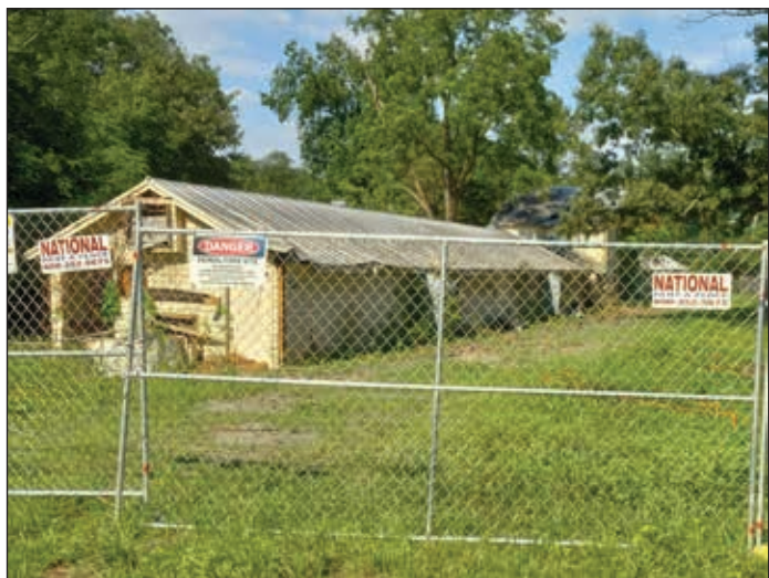
Among the buildings to be demolished are some poultry houses.
