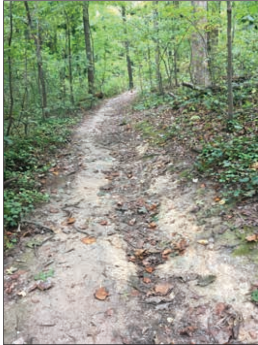
The old trail is compacted by usage and eroded by run-off from rain.
