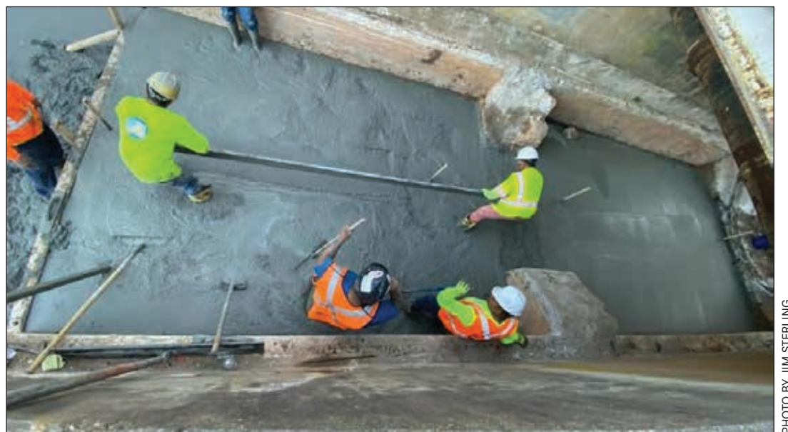
Workers pour concrete at the Lake dam.
