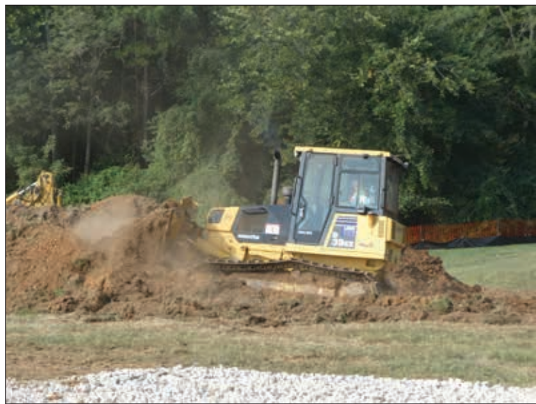
Construction begins on the Lake dam.
