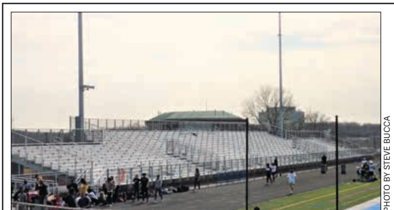
The new stadium seats at Eleanor Roosevelt High School are complete.
