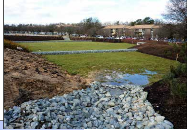
The high school's completed landscape to help prevent water pollution
