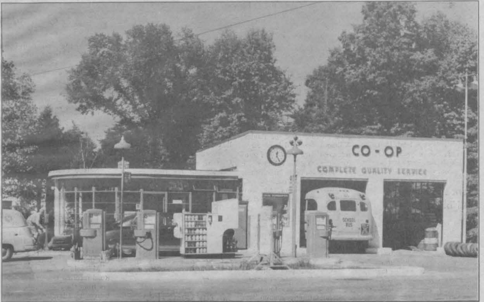
Two photographs that appear in this issue show early scenes of what is now the Mobil Gas Station on Crescent Road, opposite Gardenway. The gas station was built by the federal government in 1937 as part of the services provided to Greenbelt's earliest residents. The Friends of the Greenbelt Museum and the City of Greenbelt recently dedicated seven walking tour panels through-
