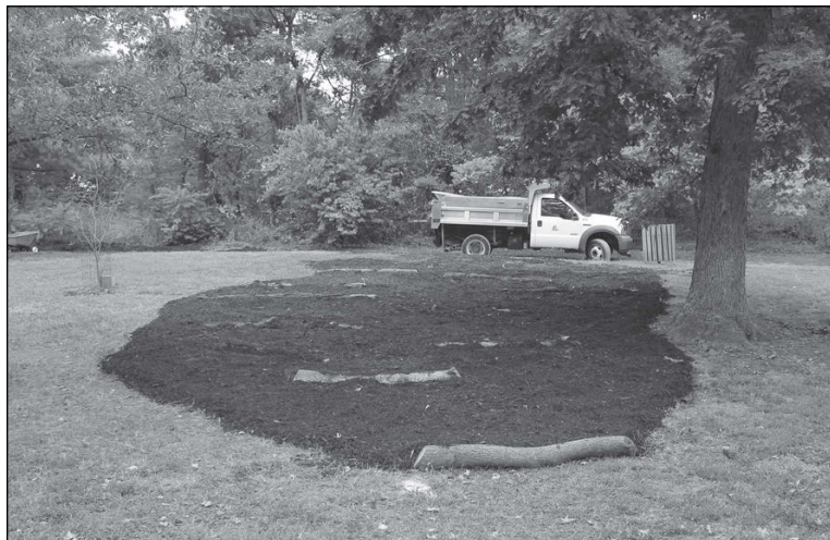
Volunteers and Public Works employees worked to build a new damming system that is hoped to slow down the flow of water over this area.
