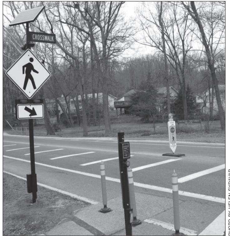
The switch located on the pole (center) activates the flashing lights mounted on the new crosswalk signs.
