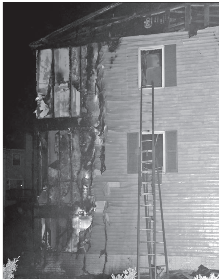
One of the badly damaged townhouses from the two-alarm fire on Jacobs Drive.
