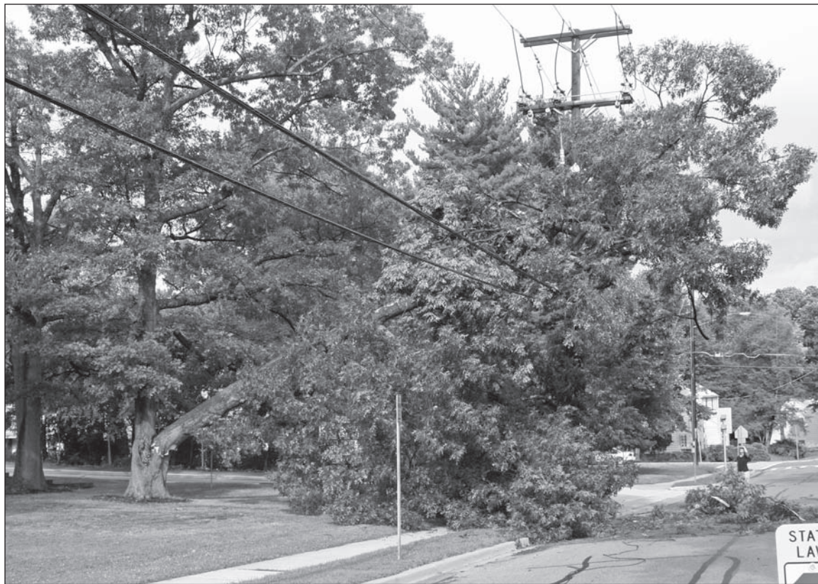
On Friday, July 31 residents of 65 Court Ridge Road saw transformer shower sparks at about 5 p.m. Then at approximately 6:30 p.m. there was a loud cracking noise and part of the large tree in front of Greenbelt Elementary School (shown here) fell onto the power lines. As a result, electricity in much of the North End was out for about two hours.
