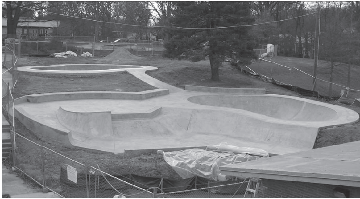
According to city officials, the new skateboard park next to the Youth Center is scheduled to open early in the new year.
