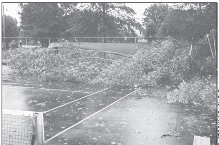
Not many residents were thinking about playing tennis in the storm's aftermath. The fence sustained significant damage when large limbs snapped from the strong winds.
