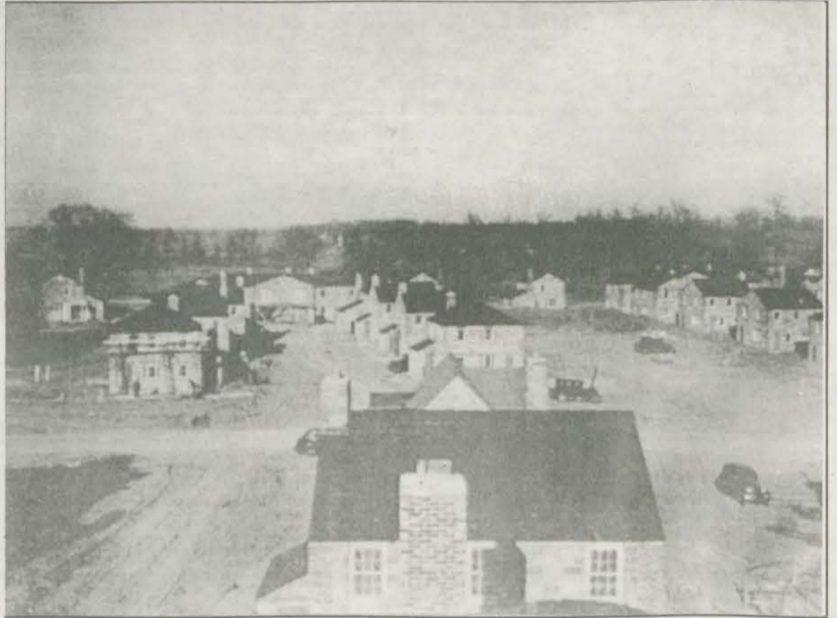
The view looking north across A section of Greendale, WI, during construction in January, 1937.
