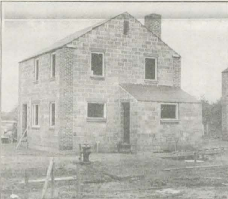
A single family house under construction on Apple Court in Greendale (October, 1936).
