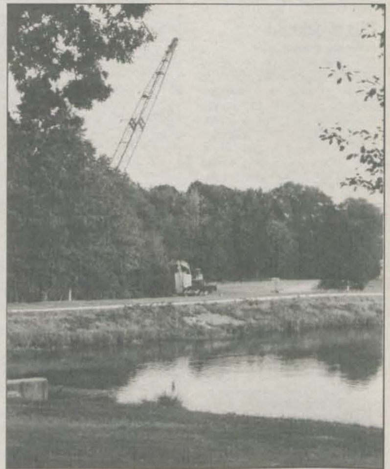
The crane looming over Greenbelt Lake shows the ongoing work on the third and final contract to repair the 96" water main.
