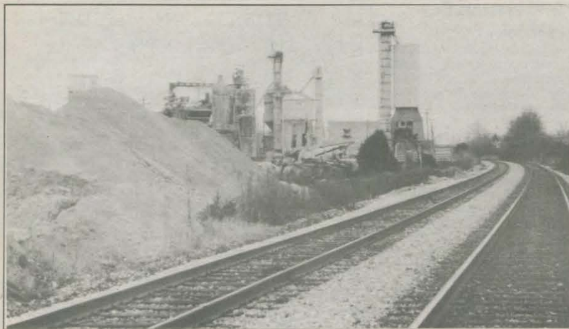
The Smith concrete plant area as seen from the CSX Railroad in 1989. Much of this facility had to be relocated or removed for the construction of Metrorail.
