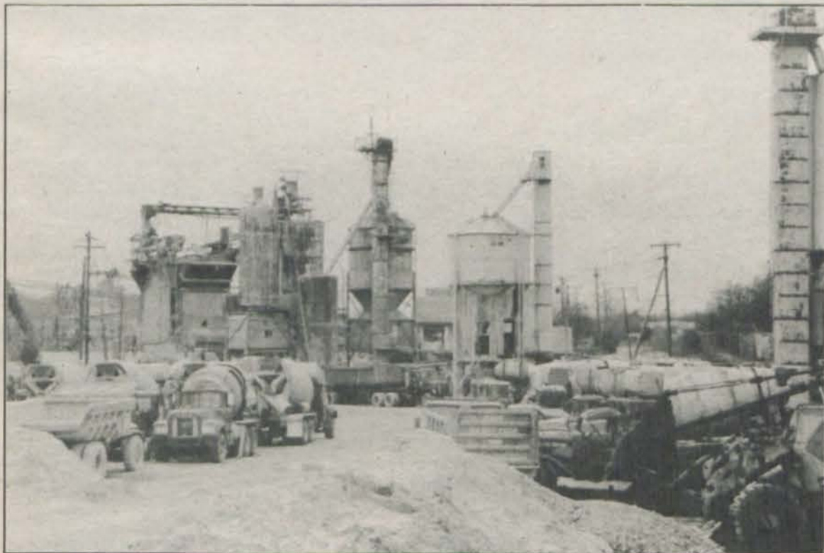
This photograph of the A.H. Smith Limited Partnership concrete plant operations area was taken by a Greenbelt citizen in 1989. Concrete is a mixture of sand, gravel, Portland cement (kiln dried limestone and clay) and water.
