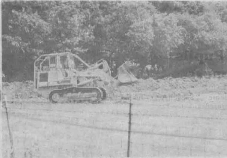
A tractor shovel moves along recently dug trench extending across part of the site behind the construction trailers. Dirt from the trench was piled beside it. —photo by Beverly Palau
