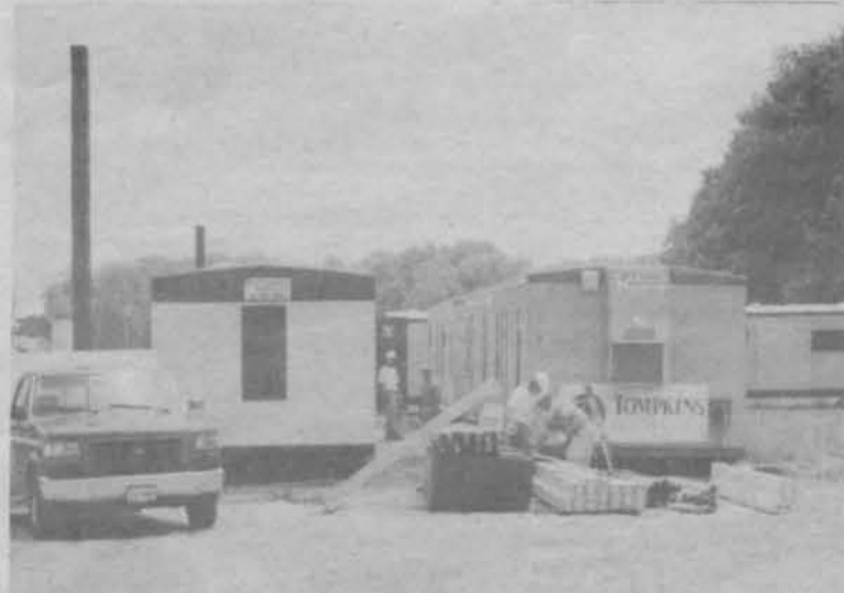
Tompkins Builders has installed its construction trailers at the U.S. Department of Agriculture (USDA) Office building site on the south side of Sunnyside Road east of the CSX railroad tracks. The builder also is doing other work. Site observers report that site work actually began before the City of Greenbelt received notice that the facility had been approved by the Secretary of Agriculture.
