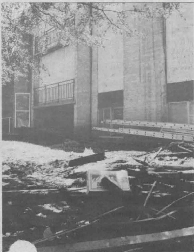
Fire damage is estimated at a quarter of a million dollars. -photo by Thelma Lore DeMola
