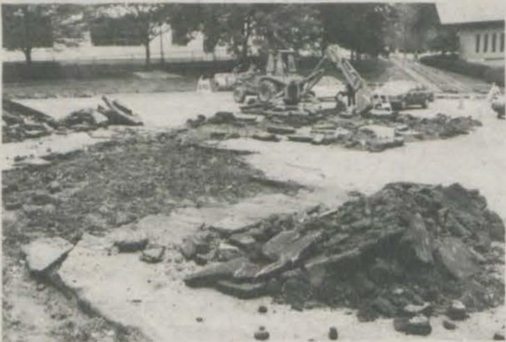
Much of the parking lot behind the library is closed for use as asphalt is torn up and piled for later removal as part of the community center reconstruction.
