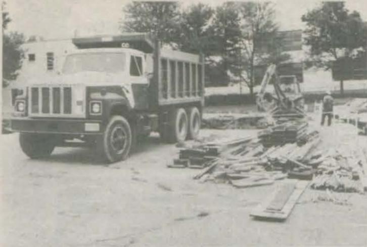
The parking areas around the community center are being reconstructed in preparation for the fall opening of the city facility. Earth moving equipment is being used to remove bad pavement and concrete. A pile of forms for pouring new concrete is in the foreground.
