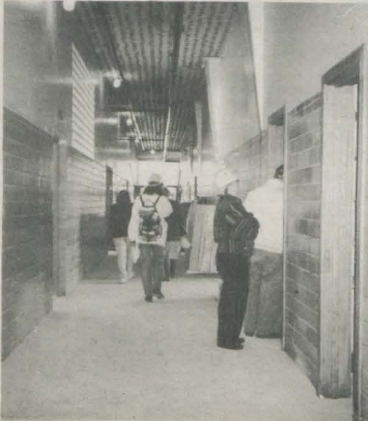
Ceramic tile remains in the old school hallways but floor tiling has been removed and new piping for a sprinkler system has been added to the ceiling.
