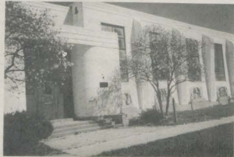
The former Center School being converted for use as a community center by the city has received a fresh coat of paint. Work still needs to be done on refurbishing the windows and doorways.
