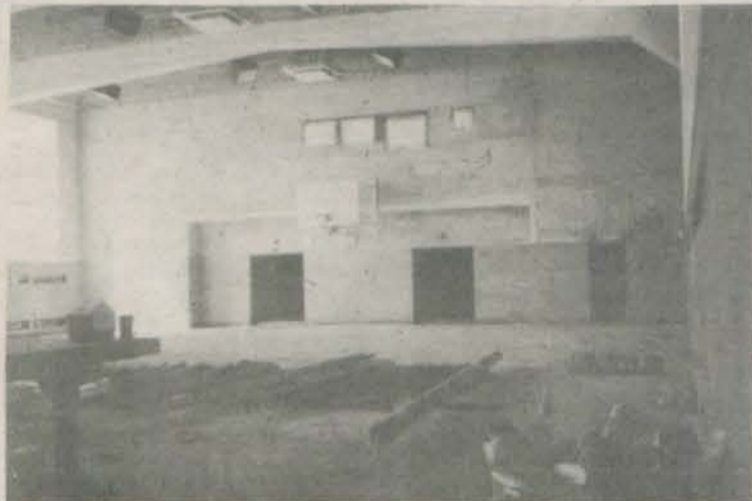
The gymnasium walls have been stripped of sound insulation and floor tiles removed.
