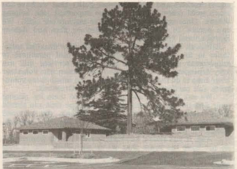
The two buildings at Schrom Hills Park flank the city, county and state champion long-leaved pine. The original park design was altered to preserve the tree when its presence was discovered at the beginning of construction.
