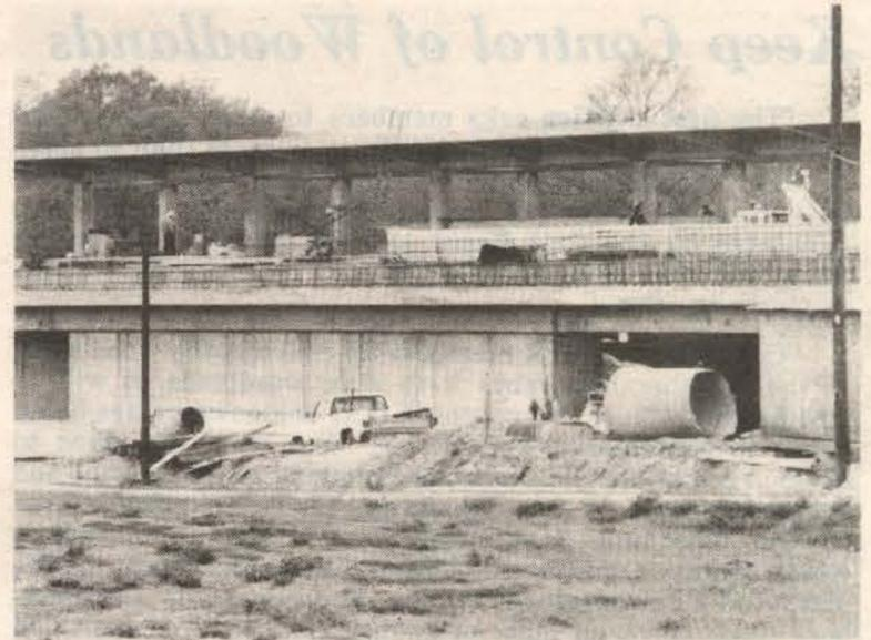
The platform canopy and track bed take shape above the mezzanine entrance to the Greenbelt Metro station. The entrances, from the parking lots and bus stops, will give access to the fare card machines and Metro center platform and, via a pedestrian underpass, to the MARC station adjacent to the Metro station. —photo by J. Henson
