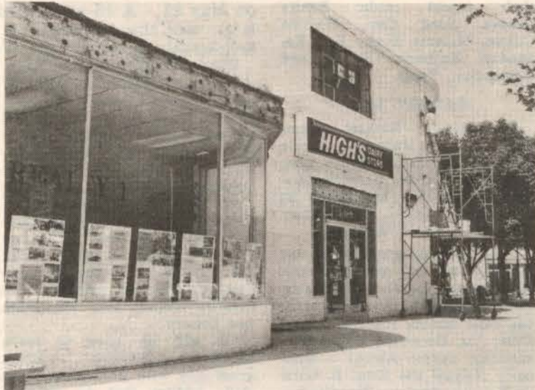
Up on the scaffold, a worker repairs the exterior of the High's store in the Roosevelt Center. — photo by J. Henson
