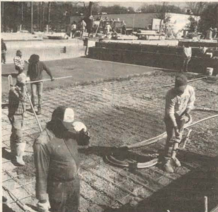
The concrete floor of the natatorium pool is poured over the rebar grid.
