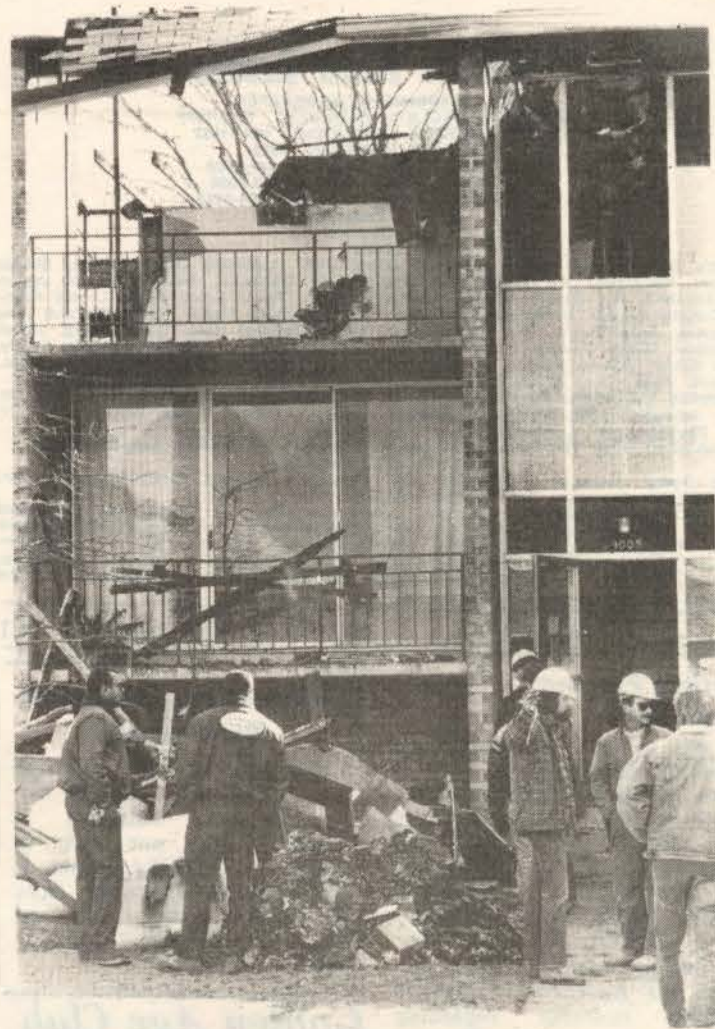
Fire that damaged most of the apartments in two adjoining buildings began on the top floor at 9005 Breezewood Terr. Springhill Lake employees were out in force Tuesday morning to begin the cleanup. —photo by J. Henson
